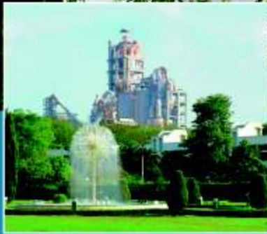
Jaypee Cement Complex, Rewa Madhya Pradesh
